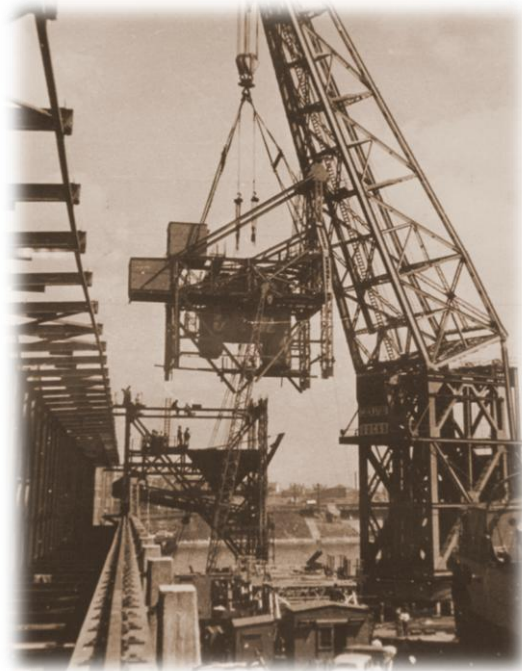
First bulk unloading used the coal crane, then 'Stothert & Pitt' gantries erected with Titan floating crane in Oct 1954; Bulk handling fully operational from 1955
