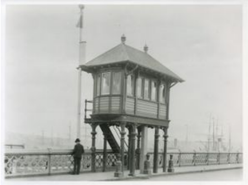
Pymont Bridge Control House in 1902
