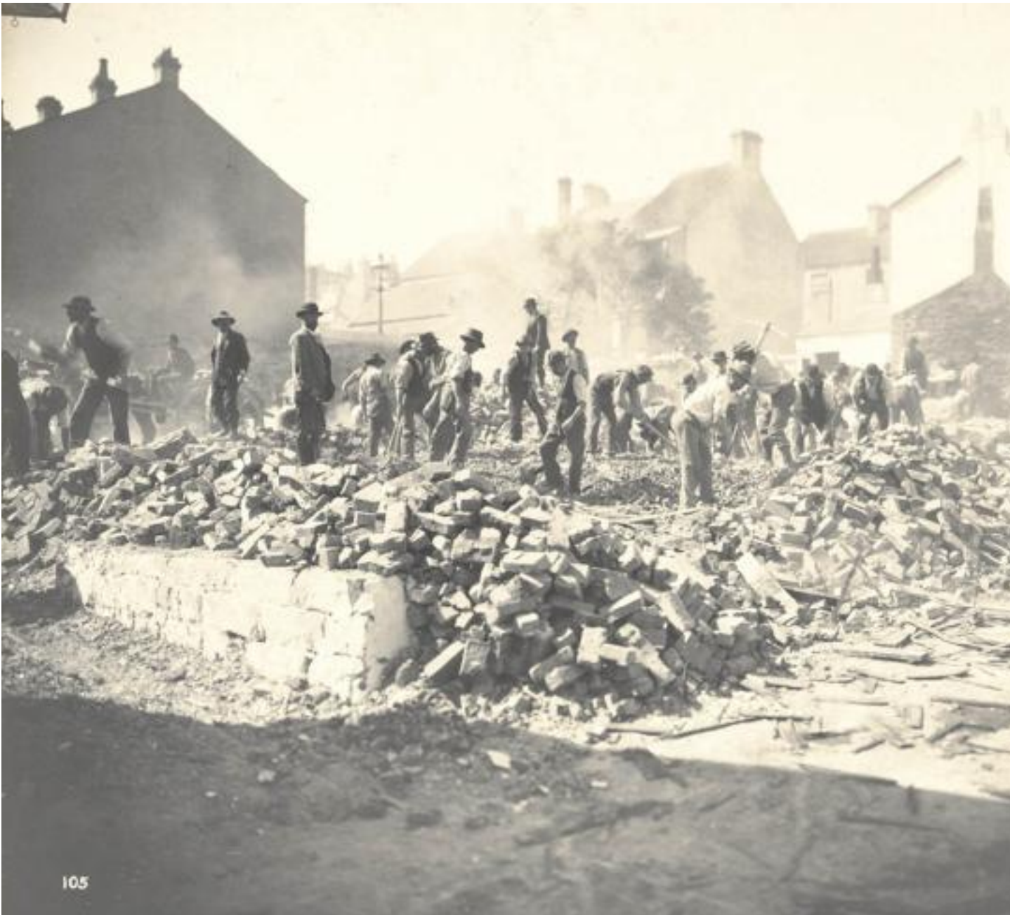
Exeter Place being demolished in 1900 during the plague outbreak. Picture: State Library of NSW
